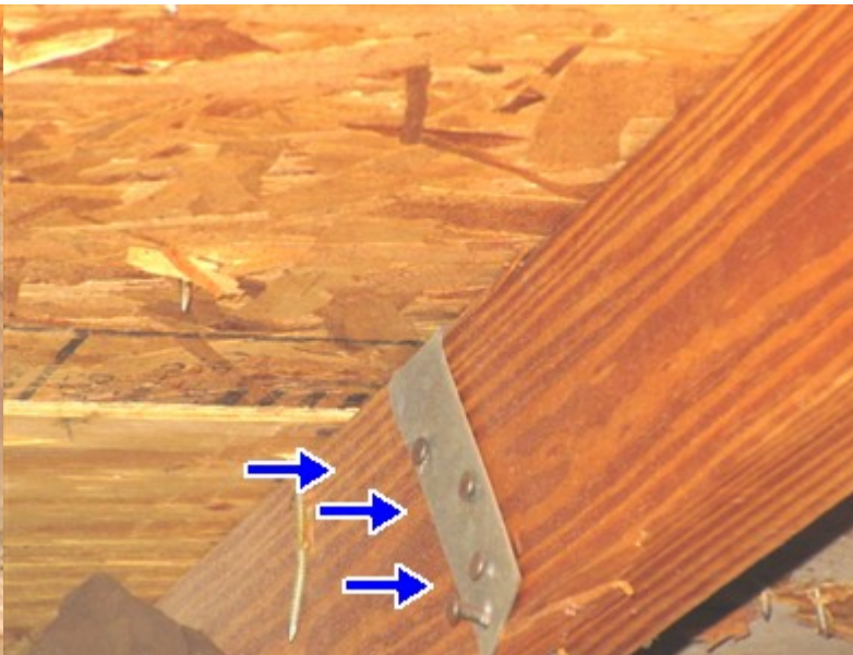
WALL TO ROOF CONNECTION
